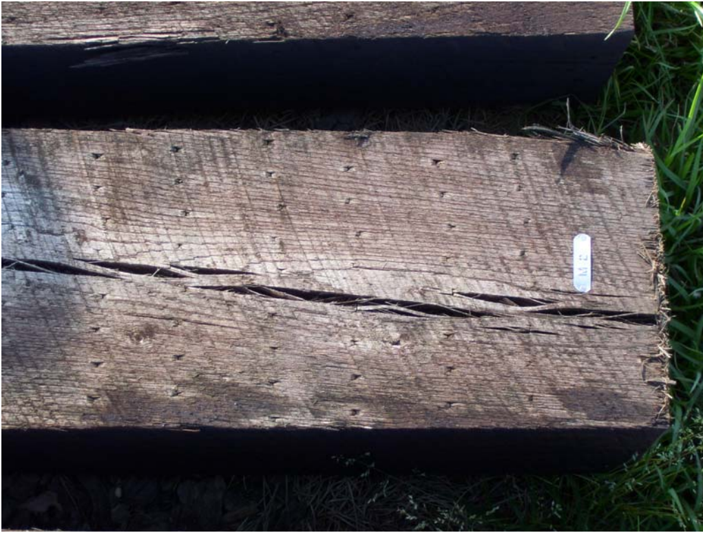
Figure 6 - Tie #2 with fairly severe checking.
